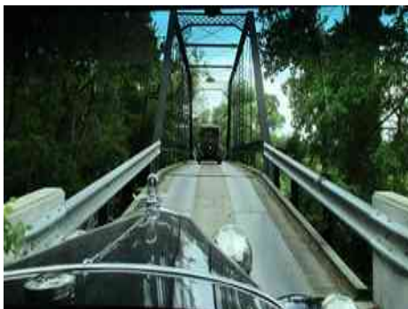
Narrow 1 lane iron bridge.
